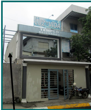
One exposed side shown here
